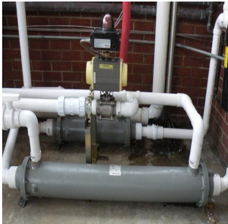
Figure 28 Heat exchangers for control of air conditions on FI test stand
